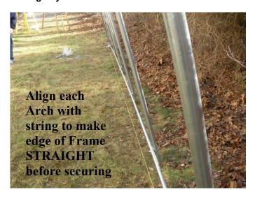
**Step 8**. Once frame is square and properly supported, tighten carriage bolts on all frame members, except for End Arch members to Cross Rails along base, side, and top. Support End Arch feet with patio blocks or bricks as needed if ground is soft and will not support weight well. After hardware is tightened, insert plastic end plugs 1-5/8" EP-1000 & 1" EP-1001 into all open ends of frame members.
