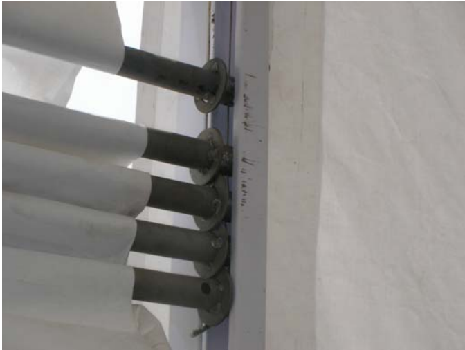
Door Tubes Inserted Into Door Track
